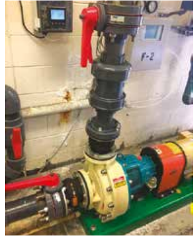
USA, Chemical plant - Caustic soda transfer
