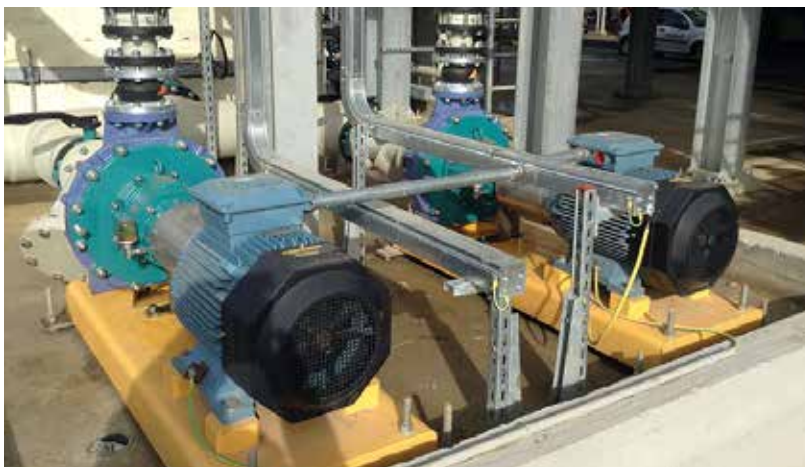
ITALY, Desalination plant
